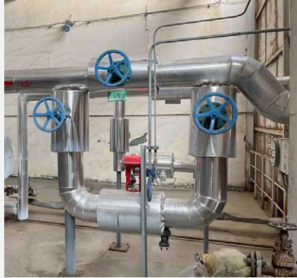
Medium-pressure steam to low-pressure steam retrofitting project
