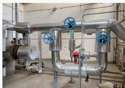
Medium-Pressure Steam to Low-Pressure Steam Technical Transformation Project
